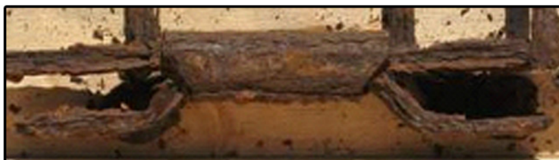
Detail of the spalling rust on a cleat. After over fifty years in a damp saline environment, a large area of the grating is in this condition.
